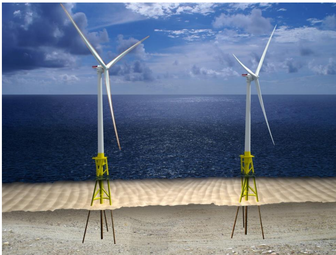
Figure 2: Artist’s rendition of VOWTAP turbines. Relative location depicted is conceptual; actual distance between turbines is likely to be between 6 and 12 rotor diameters, with tower centers between 600 and 1,200 meters apart. By comparison, an OCS sub-block is 1,200 m on a side.
