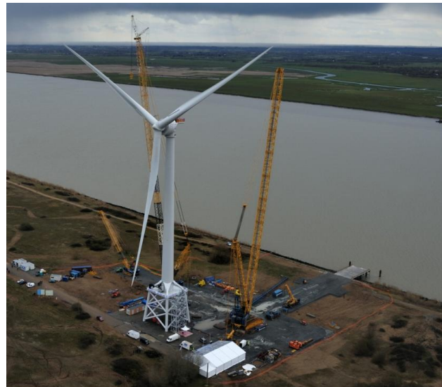
Figure 3. First HALIADE™ 150 Prototype Fully Assembled on 18 March 2012 – Le Carnet, France
